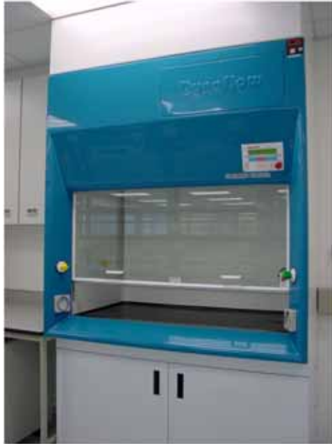
Figure 1: A conventional fume cupboard with variable air volume control
